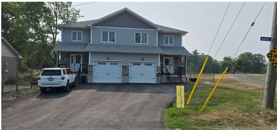
View of the existing semi-detached dwelling at 200 Maple Street North
